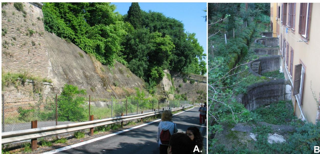
Landslides along the left side of the Tiber river valley, due to slow movement of the Pliocene clays . A. The external wall of Villa Sciarra collapsed in 1990. B. The edifices at the base of Monteverde hill have been built with horizontal arcs to prevent the effects of decompression of the overconsolidated Pliocene clays.
