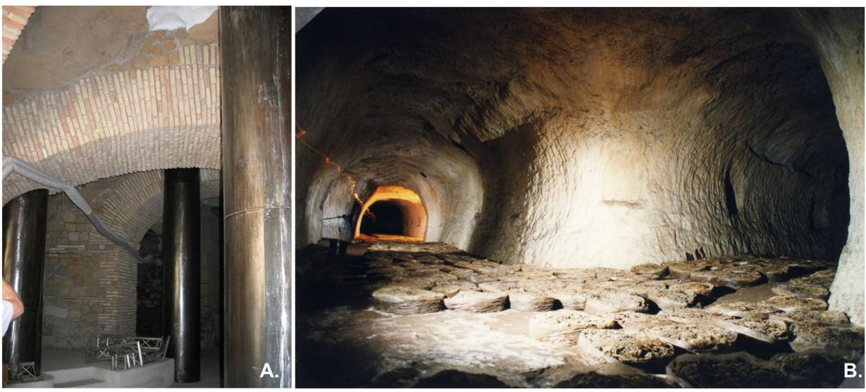
A. Tunnel excavated in the Tufo Lionato at Monteverde originally to extract building stones, have been re-inforced and longly used. Note also the vertical pole-foundation which have penetrated the tunnel from overlying constructions; B. Underground cavities used for mushroom-growing.
