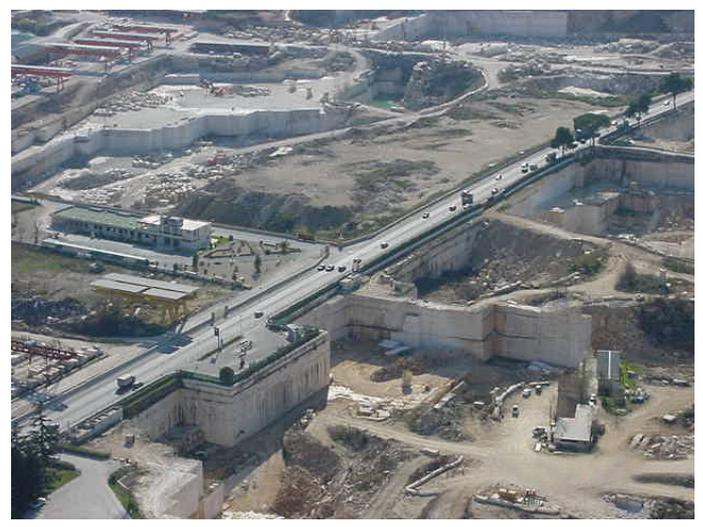
The quarries of Tivoli travertine have left a superelevated strip on which runs the Tiburtina road.
