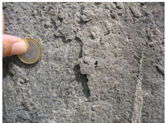
Example of weathering forms affecting Vesuvian lavas: exfoliation, Via del Sole (Naples).
