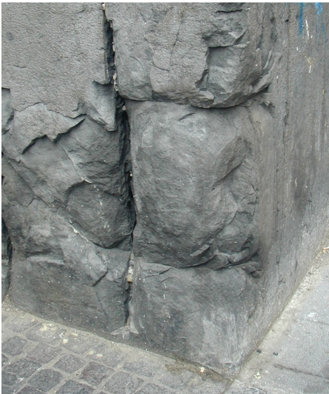
Figure 62. Weathering of the Vesuvian lavas.
