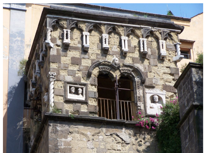
Belltower of Pappacoda Chapel (1415, restored in 1772) made with NYT, Campanian Ignimbrite and Piperno.
