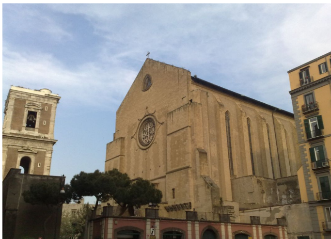
Figure 18. The Neapolitan Yellow Tuff as a building stone.
