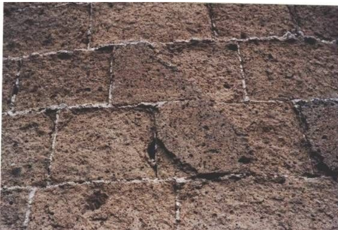
Casertavecchia Castle Mastio, example of disaggregation and alveolization in the yellow facies of CI (LYT).
