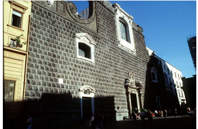
Gesù Nuovo Church. The façade of this building (begun in 1584 and completed in 1601) is of Piperno ashlar.
