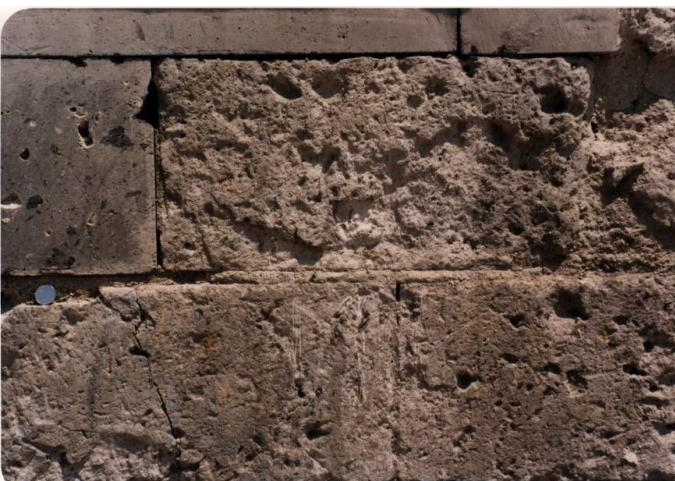
Casertavecchia Castle, example of alveolization in the grey facies of CI (WGI).
