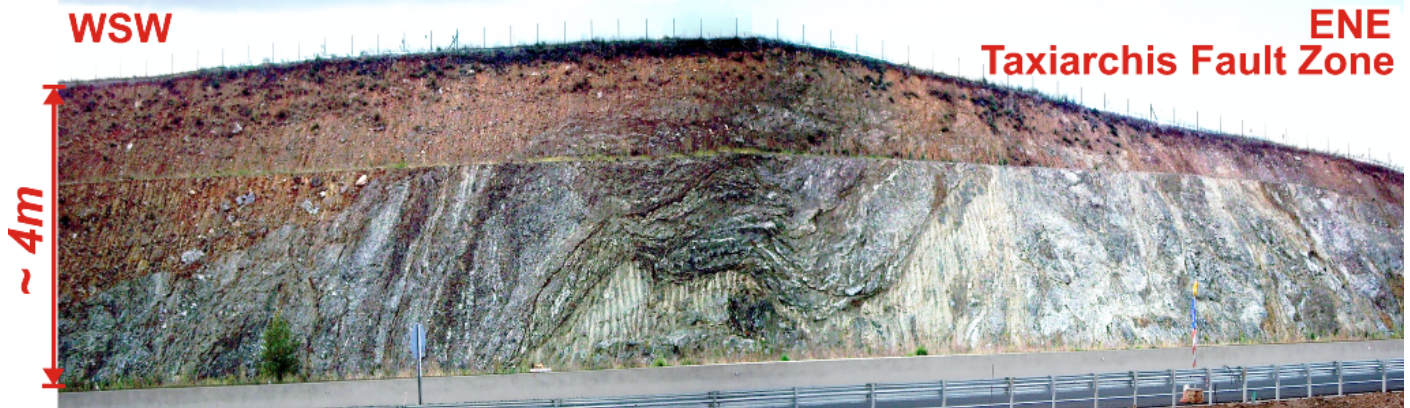
Road-cut exposure of Taxiarchis fault along Egnatia Highway.
